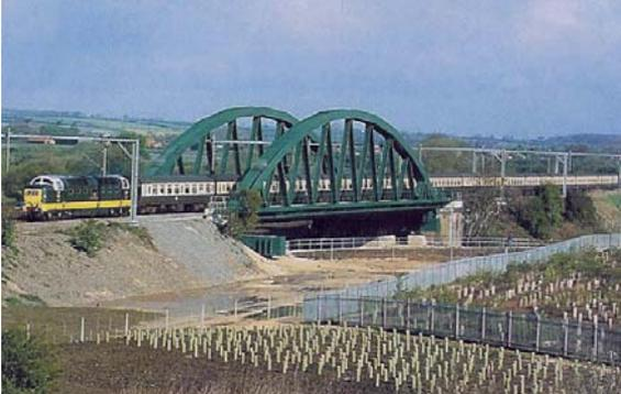
In conjunction with British Rail engineers, bridge replacement was a task that entailed precise preplanning and timing in order to demolish the existing structure and roll in place the replacement prefabricated structure, lay ballasted track, all between the hours of the last scheduled train through and the first early morning traffic.
